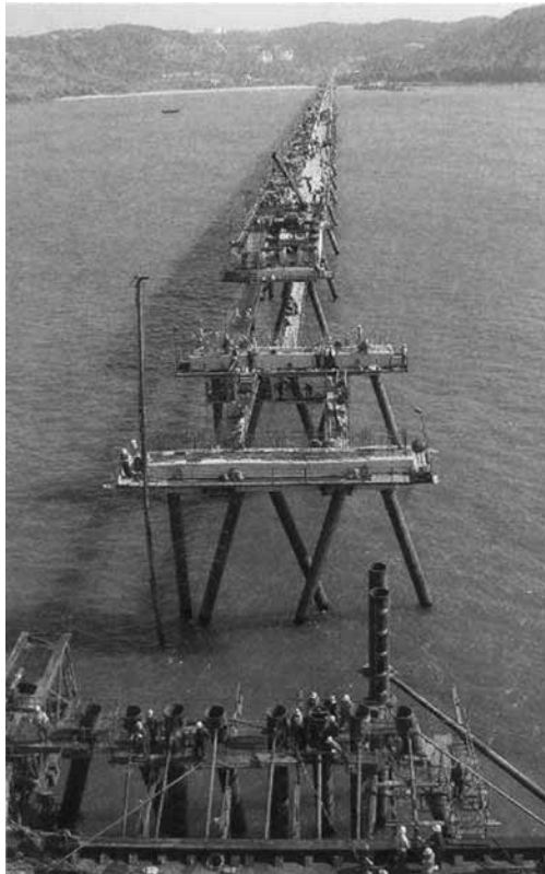
Figure 1.1 Typical exposed jetty under construction (Courtesy BeSix–Kier)
