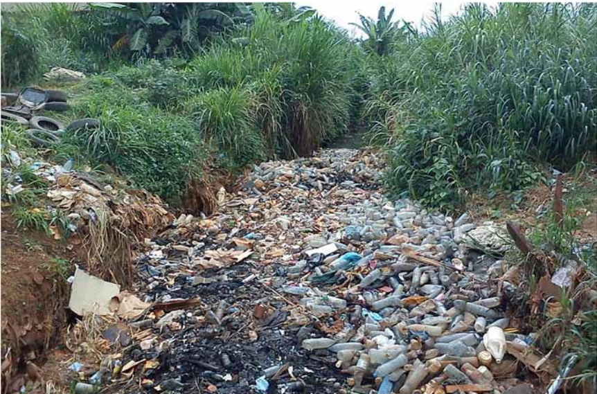
Fig. 1.1. A Choked Stream in Yaounde (Cameroon) as an Example of an Urban Hazard.
