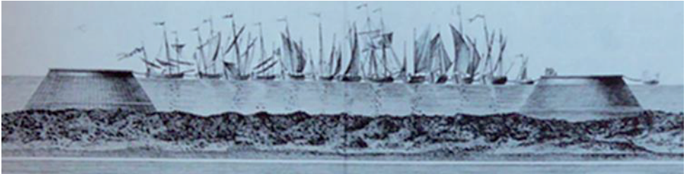
Figure 2 Use of timber cones at Cherbourg
