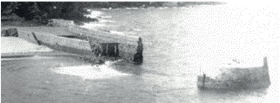
Figure 3 Failure at Greve du Lecq, Jersey, 1884
