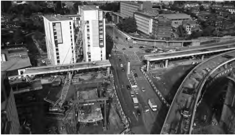
Figure 1.8 Removal of Liverpool's condemned Churchill Way flyovers [22]
