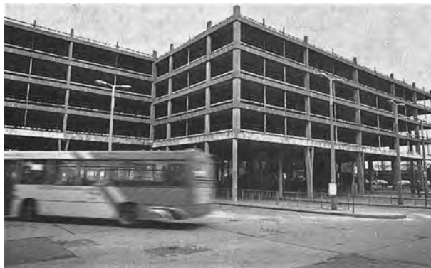
Figure 1.1 Multistorey car park in Colchester that was pulled down in 1995 because concrete corrosion problems were beyond economic repair
