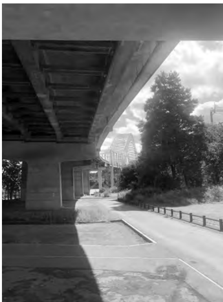
Figure 1.2 Concrete approaches to the Runcorn Bridge
