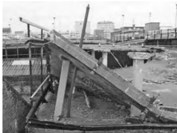
Figure 1.6 Collapse of Pipers Row multistorey car park in Wolverhampton [18]
