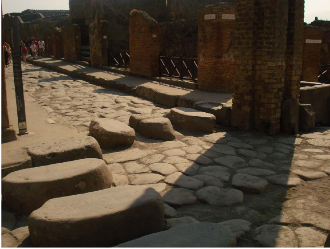
Figure 1.4 A road as a drain in the city of Pompeii (Chris Digman)
