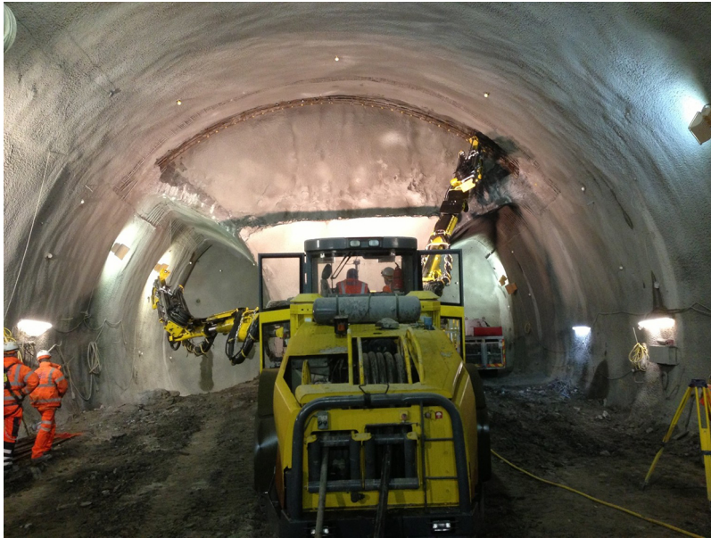
Figure 7.3 Spiles being installed with lattice girders (Crossrail Stepney Green Cavern)
