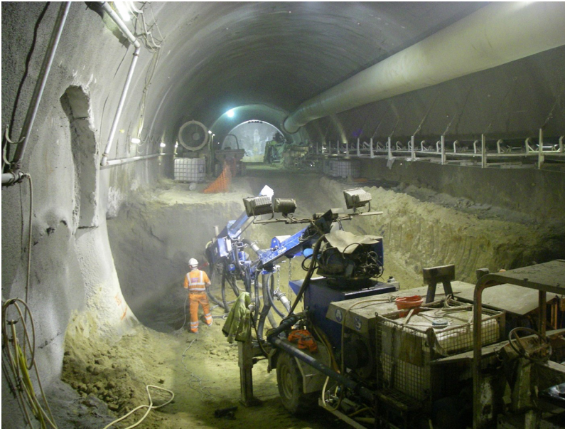
Figure 6.4 Top heading and invert separation (A3 Hindhead Road tunnel)
