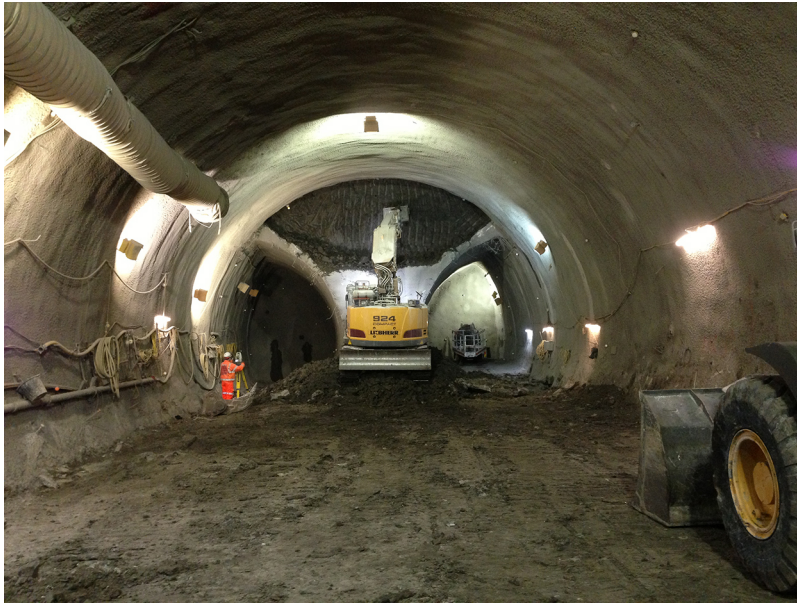
Figure 6.6 Double sidewall drift excavation (Crossrail Stepney Green cavern)
