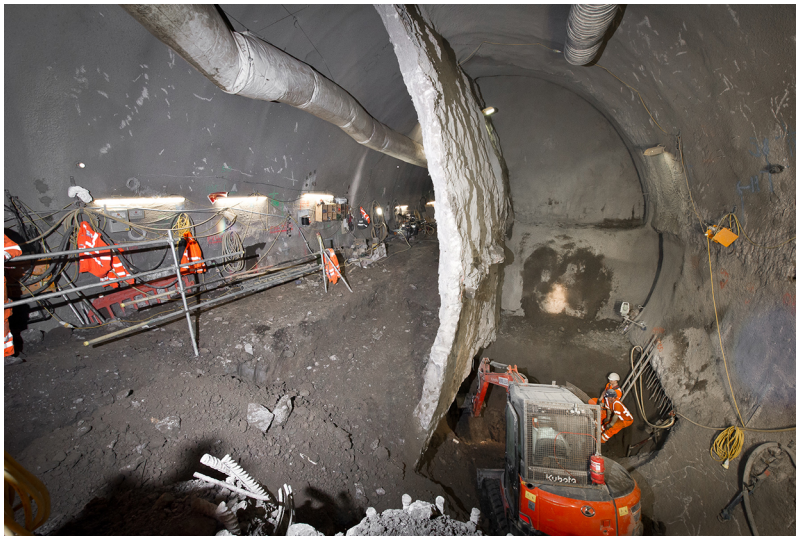
Figure 6.5 Single sidewall drift excavation (Tottenham Court Road Station Upgrade)
