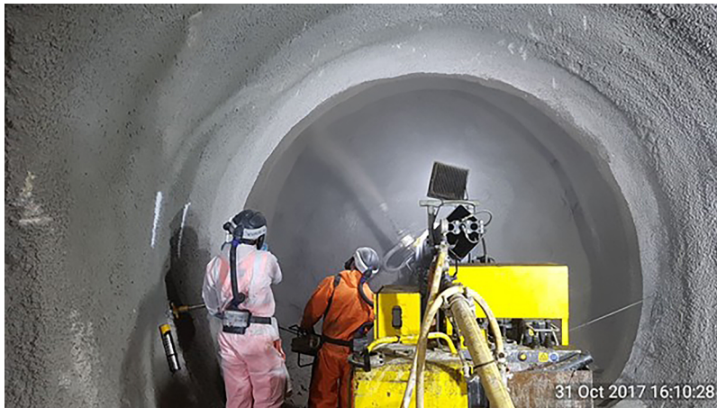
Figure 6.2 Full-face robotic lining installation (Bank Station Capacity Upgrade)
